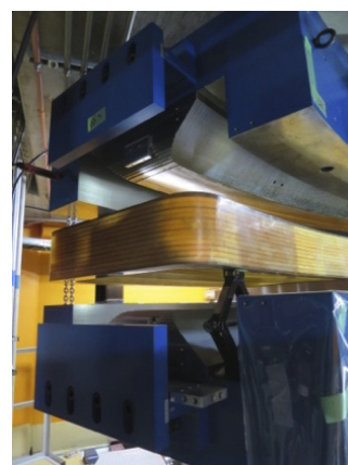
Fig. 2. Installation of new coil in DMT3 iron yokes.
