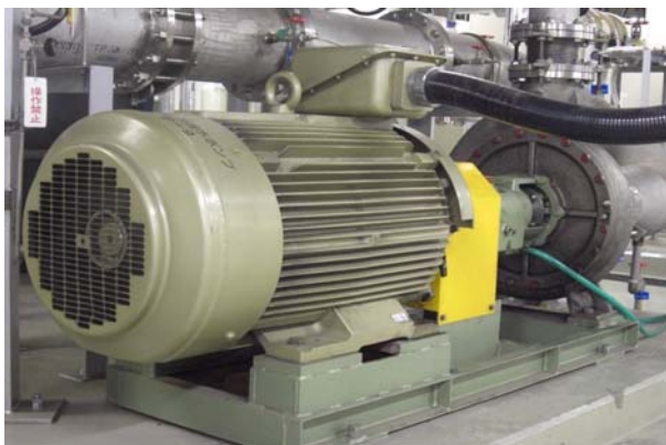
Fig.1. Photograph of the Water-pump with highly effective motor. ( JIS Standard C4212 )
